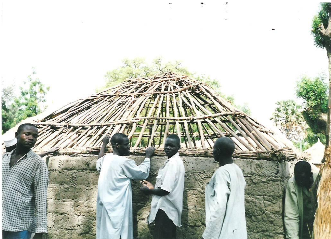
Figure 17: Making the skeletal roof to match the wall
