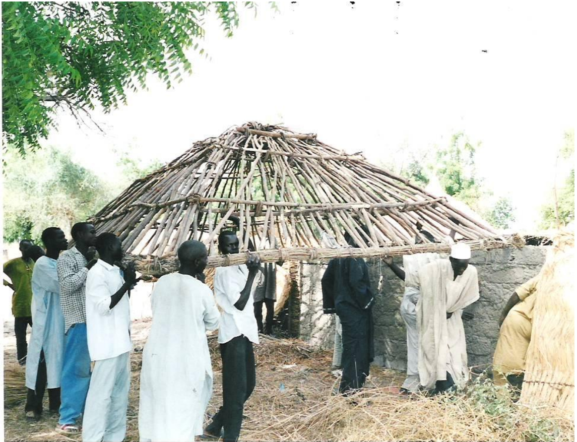
Figure 20: Lifting the roof onto the wall
